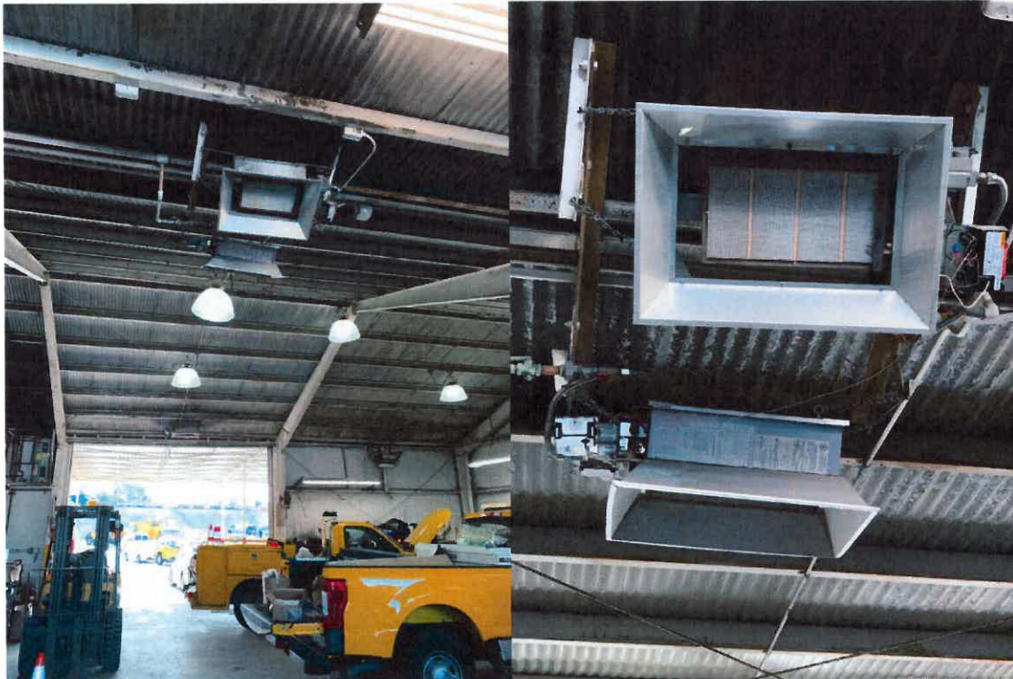
5 Photo of gas operated infra-red heaters
