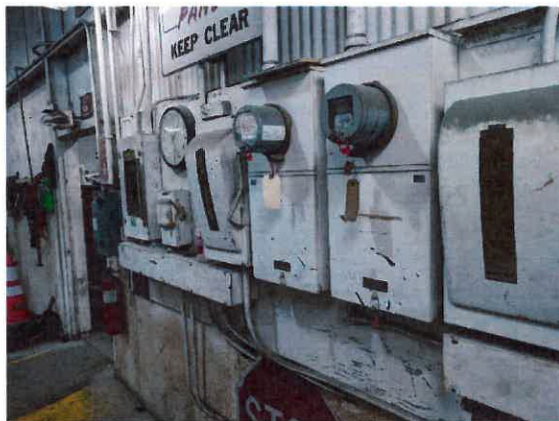
Figure 4: Utility service meters, main fuse disconnects, panels, and wire ways.
