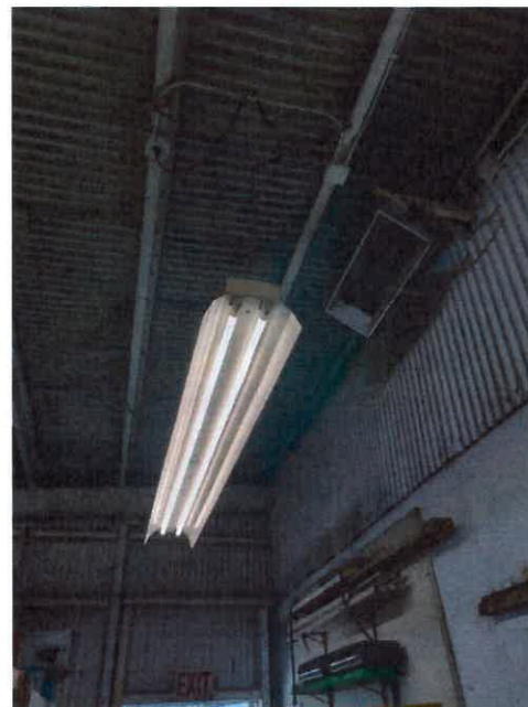
Figure 7: Exit to back of building is not illuminated properly nor is there a bug eyes light fixture.
