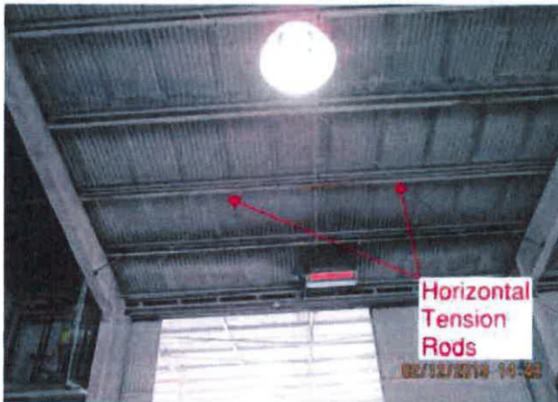
(Photo C – Horizontal Tension Rods)
