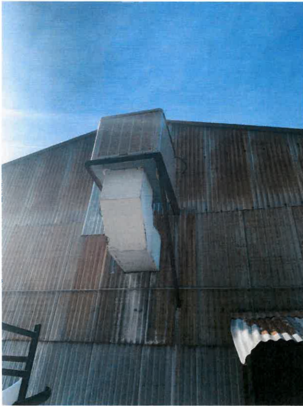
3 Photo of mezzanine evaporative cooler unit
