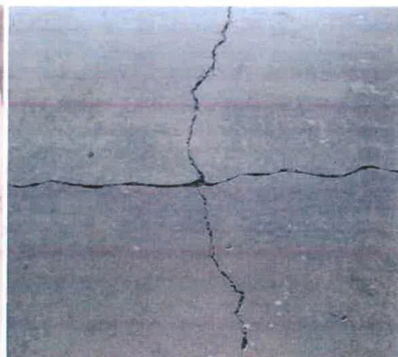
(Photo Q – Cracked Slab)
