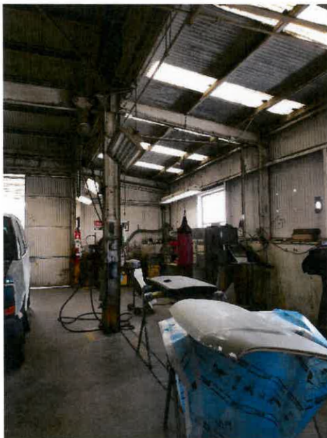
Figure 9: Not all fluorescent light fixtures are working.
