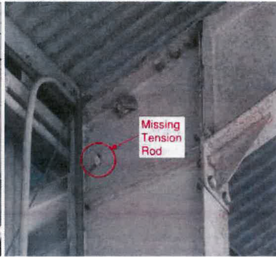
(Photo I - Missing Tension Rod)
