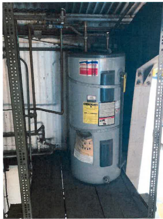
9 Photo of electric water heater
