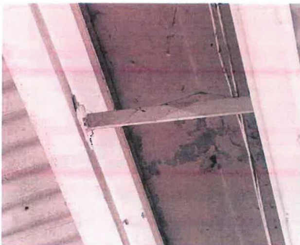
(Photo P – Possible Diaphragm Discontinuity)
