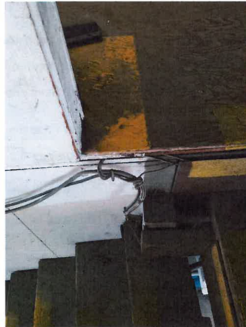
Figure 6: Exposed unsecured wires on the side of a stair case.
