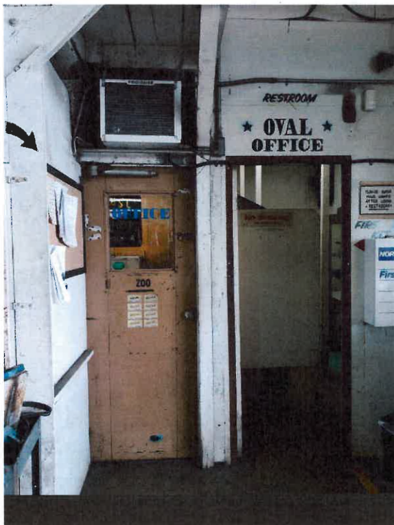
Above: Non-compliant office, restroom, and lunch room doors. Below: Inadequate and inaccessible restroom facility.
