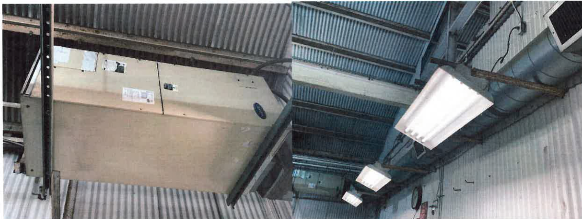
6 Photo of prep room ceiling hung fan coil
