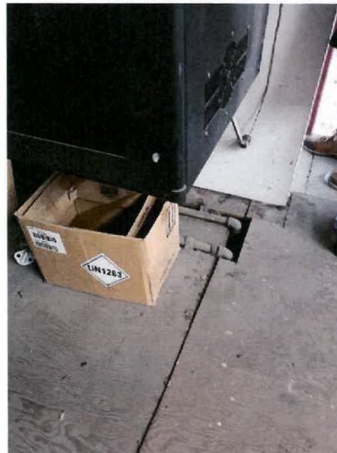
Figure 12: Communication server rack has unsecured exposed conduit going down into the floor below.
