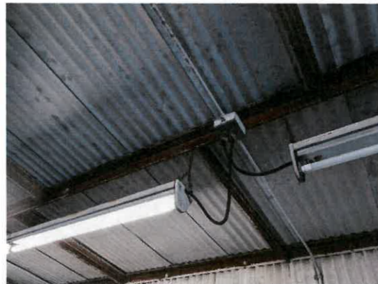
Figure 10: All fluorescent light fixtures are Plug in type.
